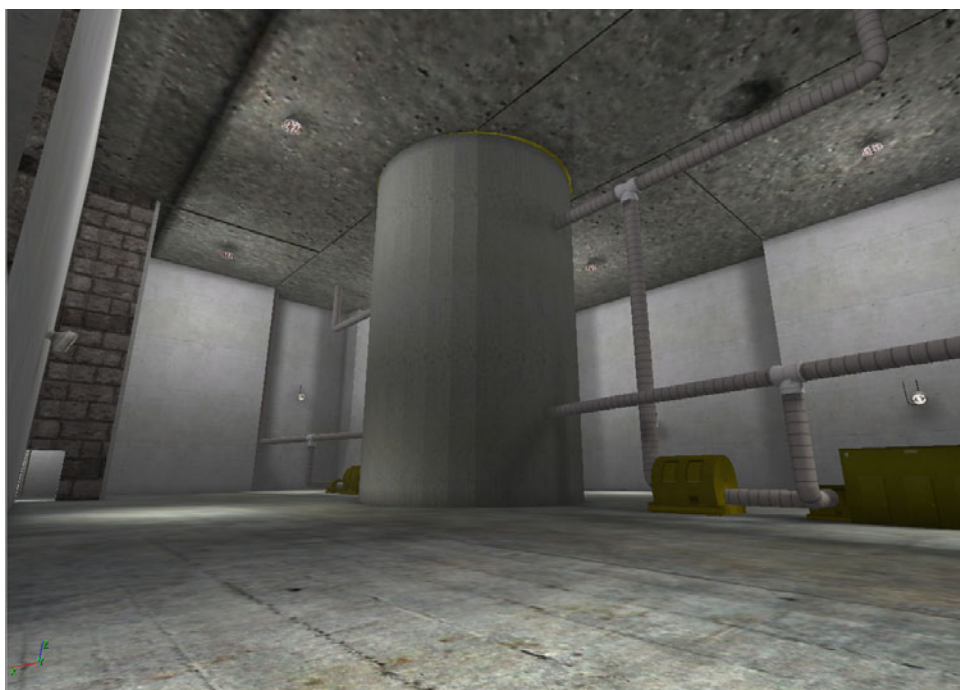
Figure 4. Exterior of Lower Portion of Reactor Vessel Showing Circulators
