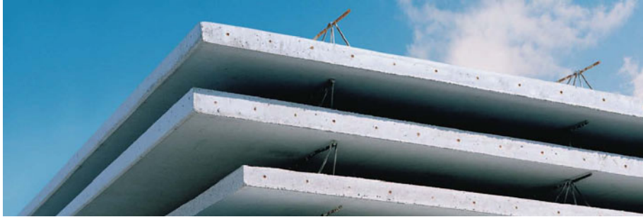
Figure 1: Sheet Piling Floors
