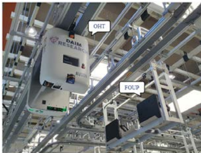
Figure 1: Components of an overhead transport system.
