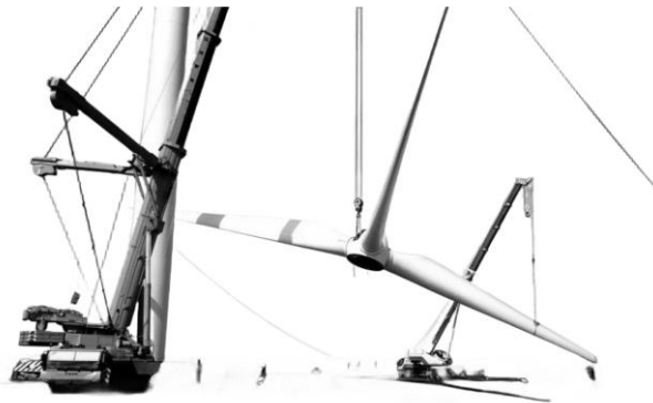
Figure 9: The blade lifting process.
